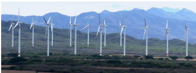
Figure 10 Onshore Wind Farm [121]
